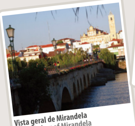
Vista geral de Mirandela Overall view of Mirandela
